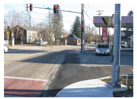
TrafInfo Communications, Inc. (TrafInfo) was responsible for the preparation of the traffic signal plans to upgrade an existing traffic signal to include a new mast arm to provide better visibility as well as emergency pre-emption.
